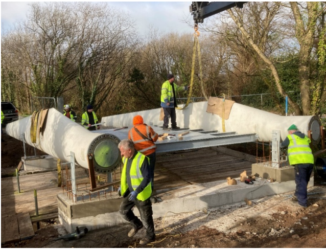
Figure 3. Bladebridge during installation on the Midleton-Youghall Greenway.
