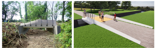
Figure 2 (a). Cork BladeBridge rendering with cut blades and exterior guardrail. (b). Cork BladeBridge rendering with full-length blades and guardrail above blades.
