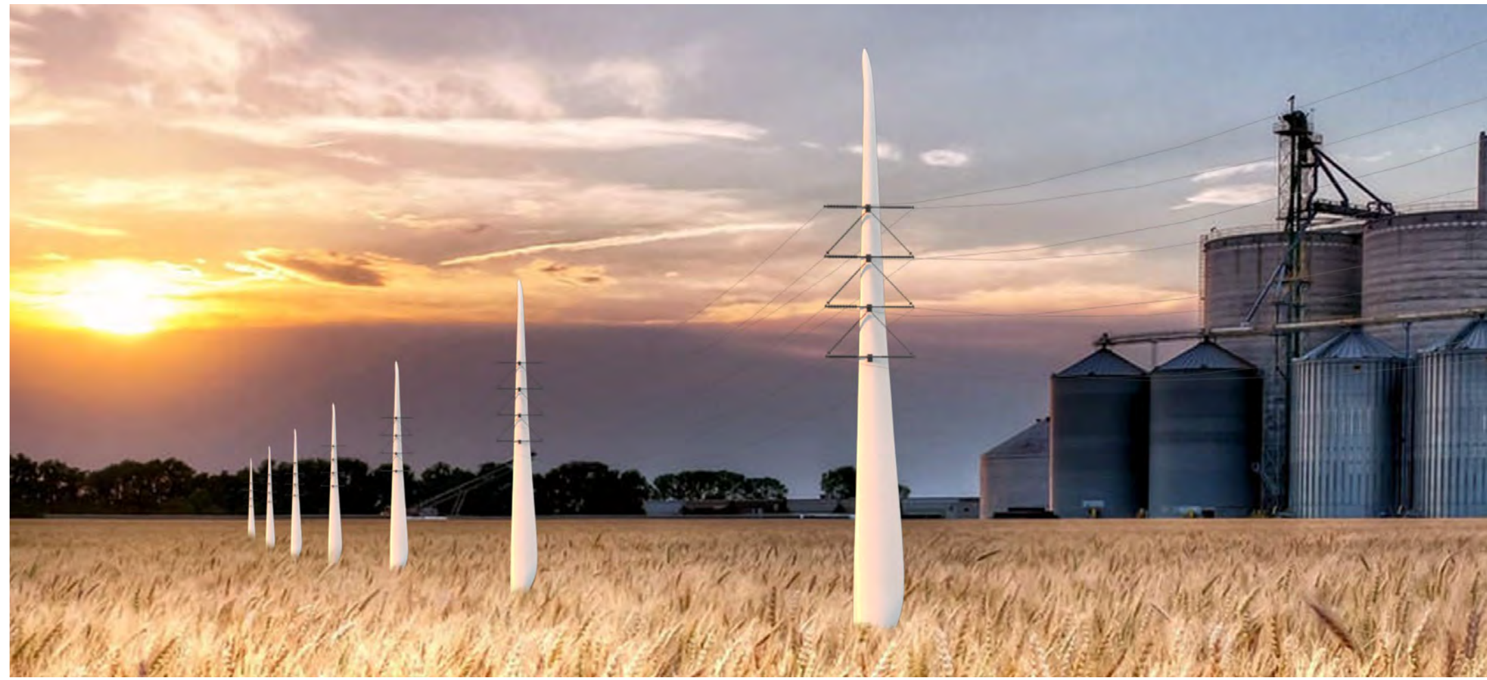
Figure 1: BladePole as a series of straight run Tangent Poles in a double circuit 230 KV transmission line
