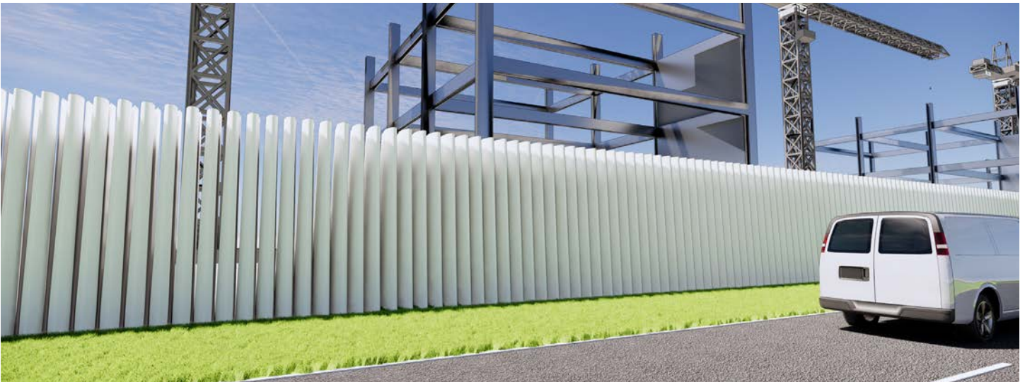
BladeBarrier from 13.4m N29 blades arranged in a regular repeated pattern around a construction site
