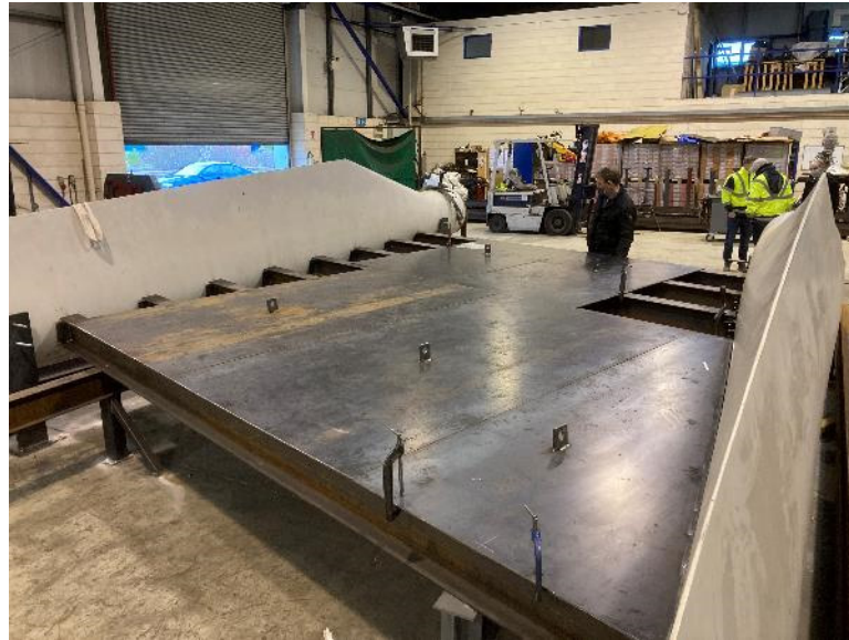
Figure 8. Fabrication and assembly of the Cork BladeBridge at the fabricator.
