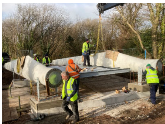
Figure 7. Middleton Greenway BladeBridge installed on site, January 2022.
